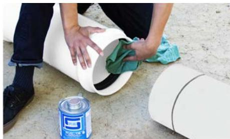
**Step 3:** Apply a lubricant recommended for PVC to the spigot end. Avoid applying lubricant directly on the gasket in the bell instead of the spigot.
